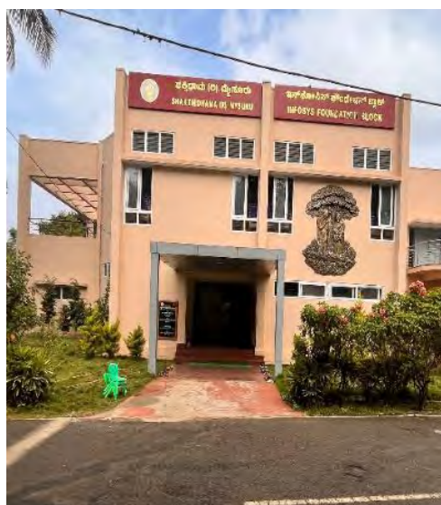
Figure 110: Infosys Foundation block at Shakthidhama
