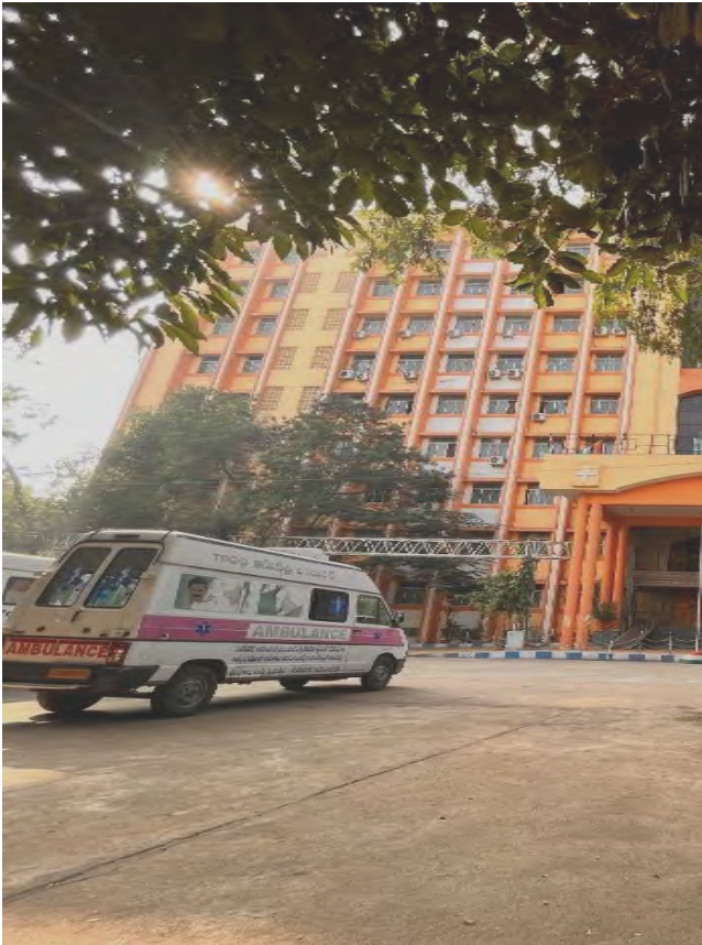
Figure 174: Gandhi Hospital, Secunderabad, Telangana
